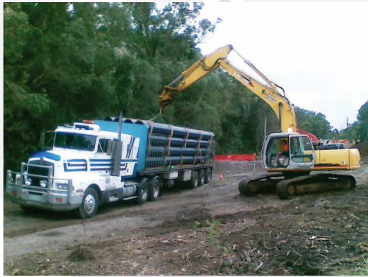
Construction of the pipeline begins
