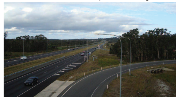
The completed Caloundra Road upgrade
