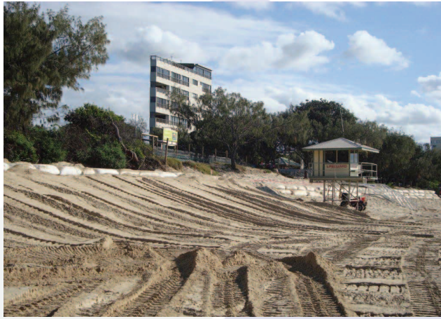
The wall of geo-textile fabric bags under construction at Mooloolaba Beach
