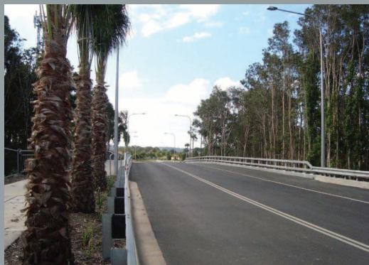
A major feature of the entrance is a bridge across Sippy Creek into the estate
